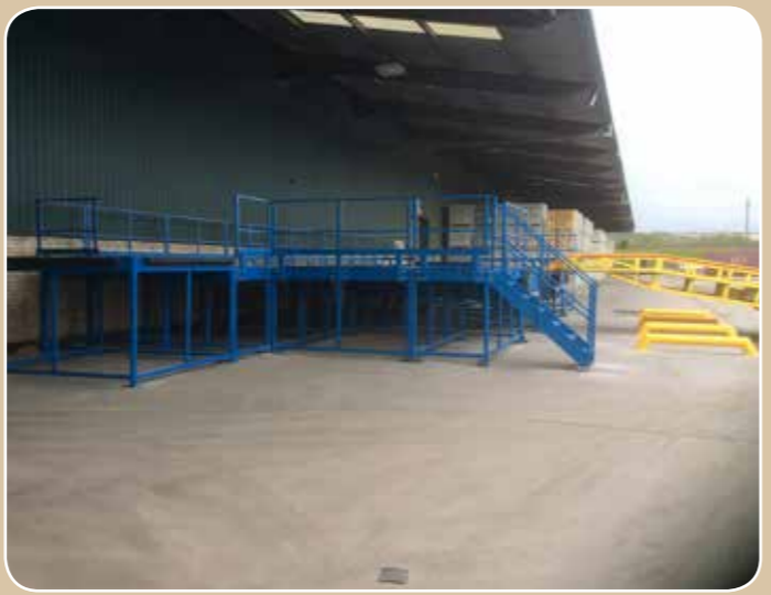
MODULAR DOCK SYSTEM GRANGEMOUTH
