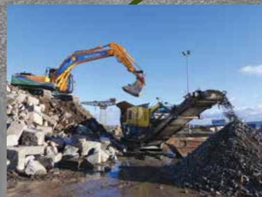
AGGREGATE RECYCLING - CRUSHER
