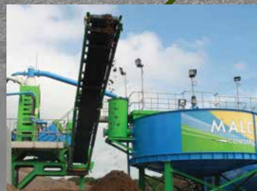
AGGREGATE RECYCLING - WASHPLANT
