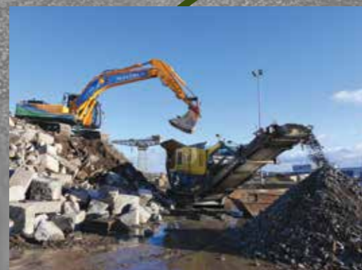
AGGREGATE RECYCLING - CRUSHER
